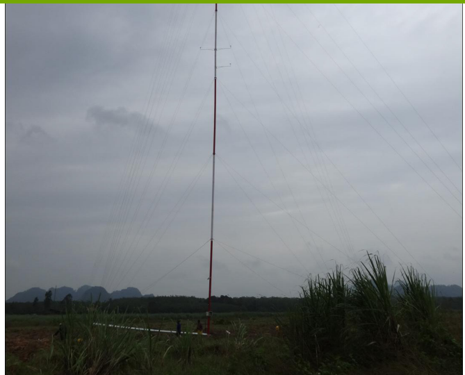
Single pole wind mast at 60m height for wind measuring at selected site
