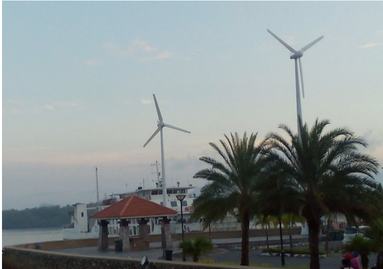
Demonstration small scale wind turbines installed at identified location.
